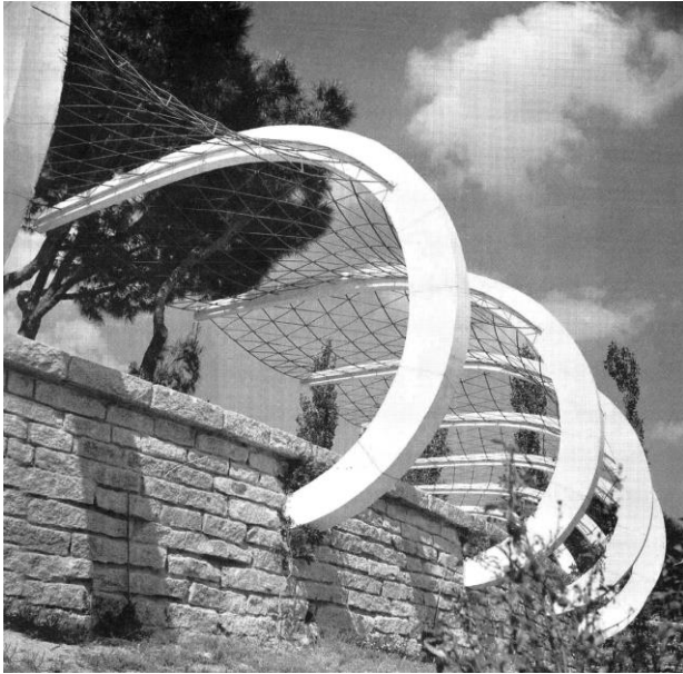
Figure 9. Cantilevered reinforced concrete pergola
